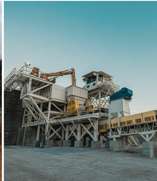
LANNON STONE Lannon, Wisconsin 3862j, 6228f feeder, 200 ton rock box
